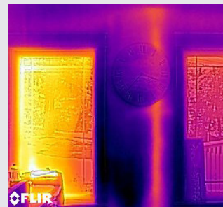
Warm Drain Pipe in Wall
